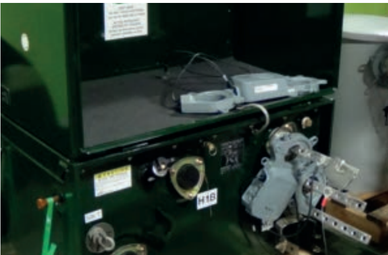
Installation of GRID 20/20 OptaNODE devices
